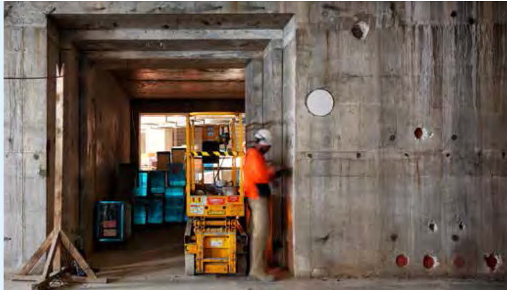
Construction of the Victorian Comprehensive Cancer Centre
