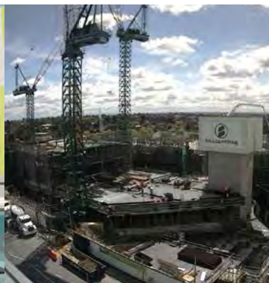
Construction of the Box Hill Hospital
