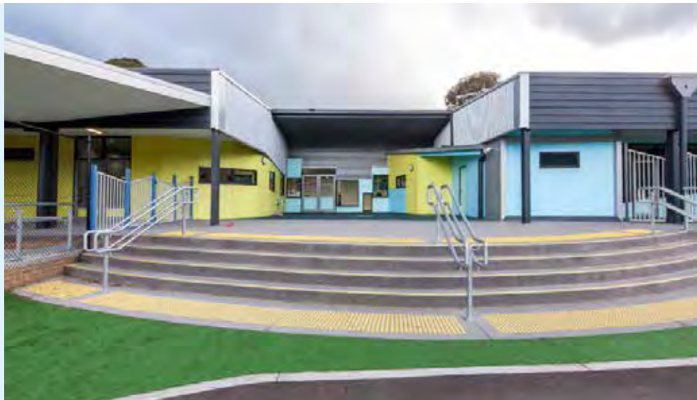
Eastern Ranges School in Ferntree Gully.
