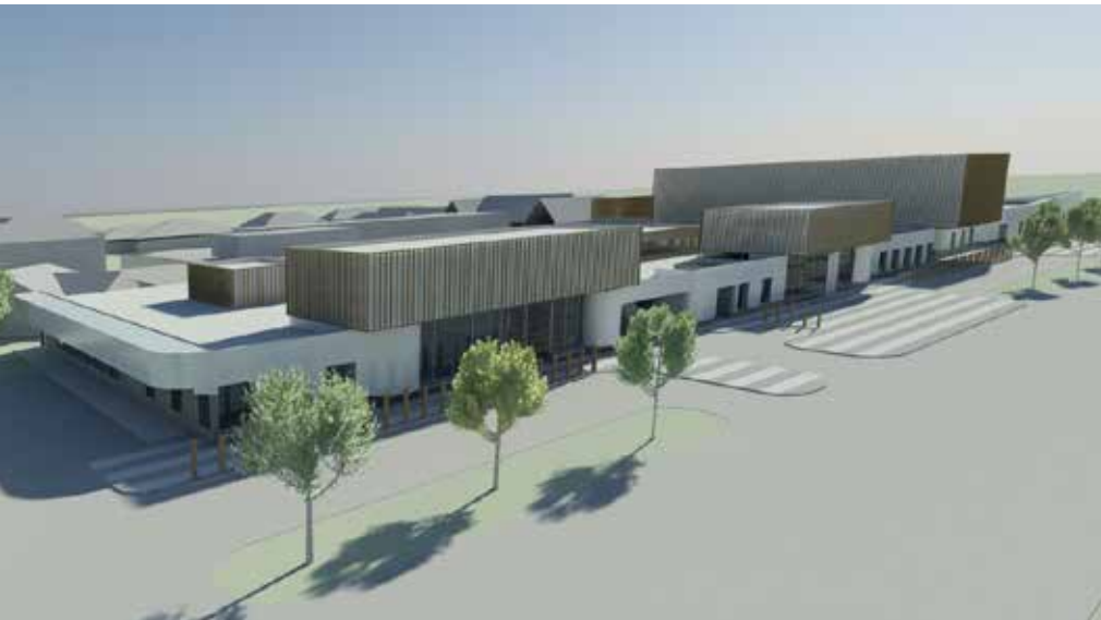
Echuca Hospital redevelopment
